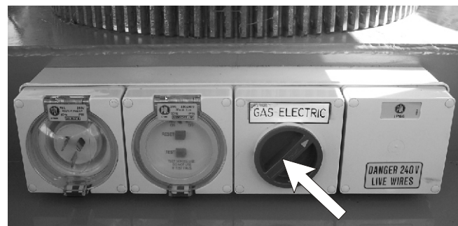
Figure 11.10 - Petrol/Electric Switch
