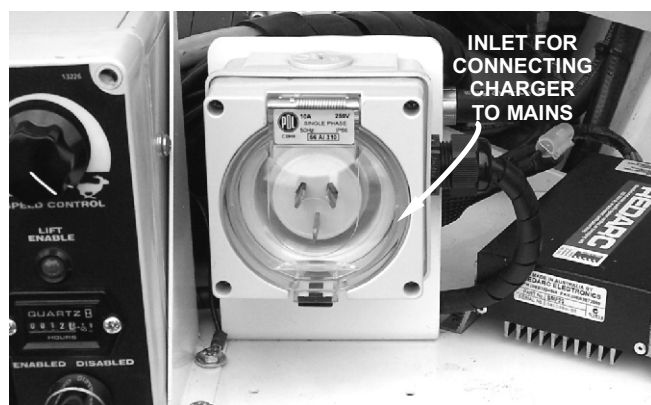
Figure 11.8 - Mains Power Connector For Charger
