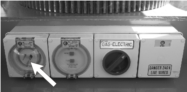
Figure 11.11 - AC Power Input Connector
